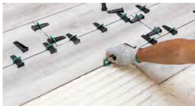
1. Colocar bases / Place the base / Placer les bases
